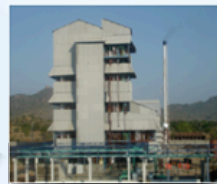
Bio Fuel Plant
